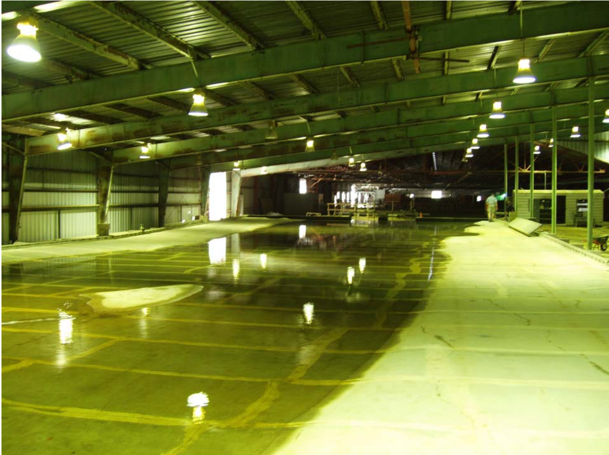
Figure 6. Tailrace (Looking Downstream from Right Bank)
