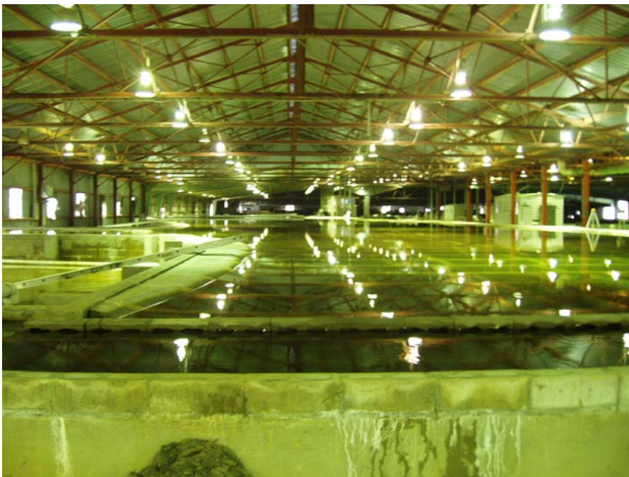
Figure 3. Forebay (Looking Downstream from Headbox)
