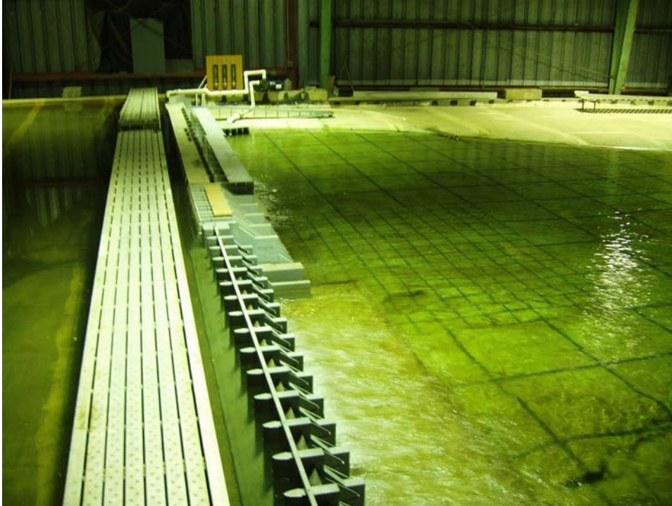
Figure 4. Spillway (Looking from Right Bank)
